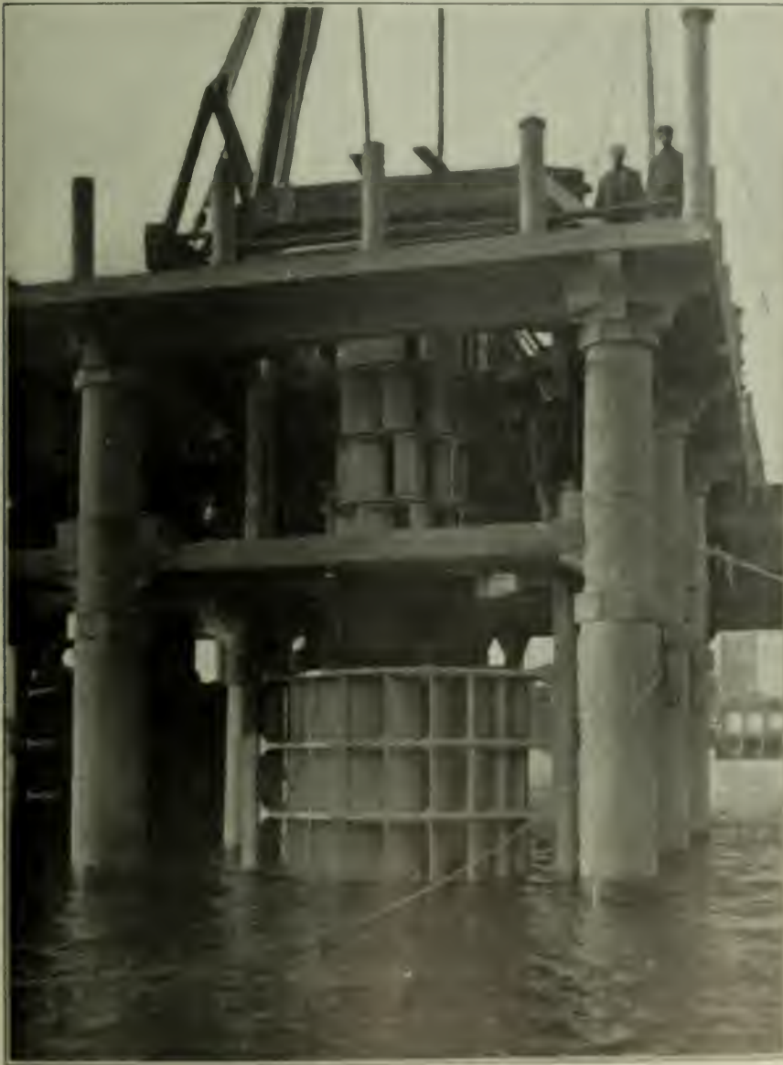
FIG. 1. SNEE WAVE MOTOR BEING INSTALLED BY STURGEON CITY
